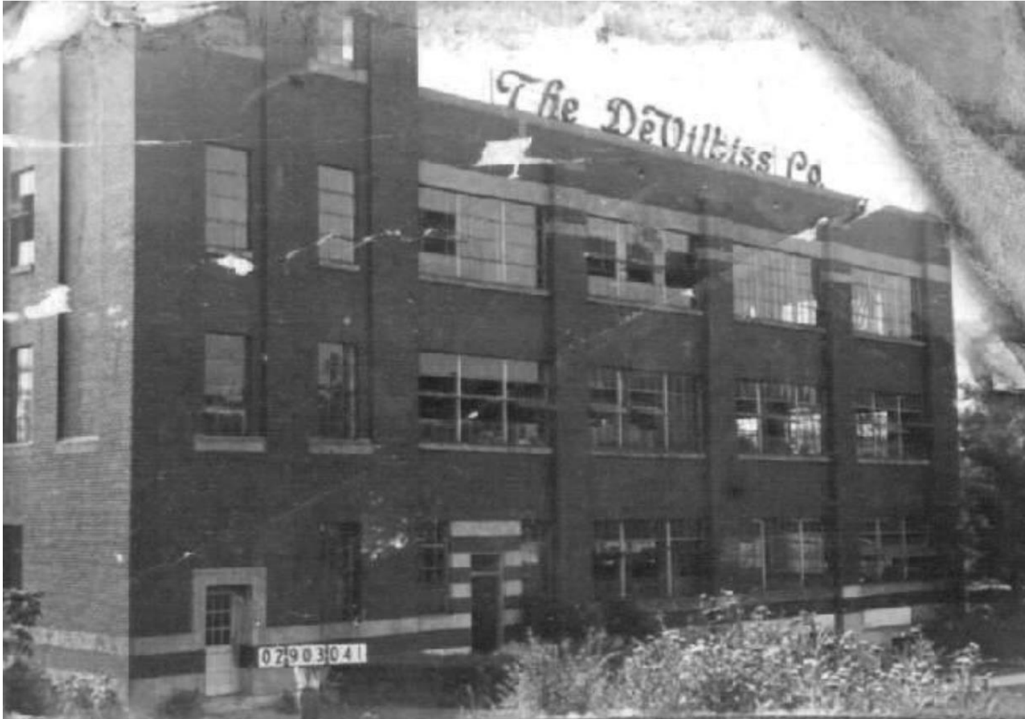
Figure 10 - 300 Phillips Ave, Block Card Photo. 1937
