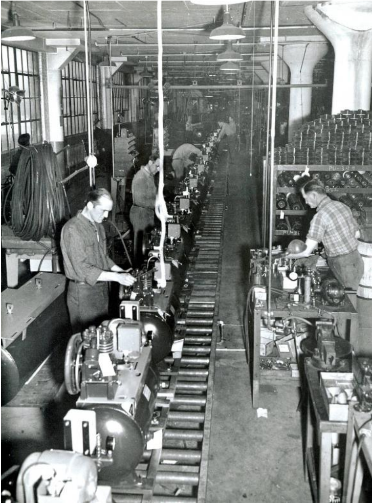
Figure 12 - Historic Photo – manufacturing, 2 nd floor
