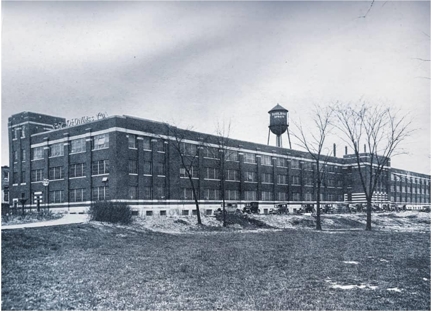
Figure 9 - DeVilbiss Manufacturing Company Building, circa 1920s
