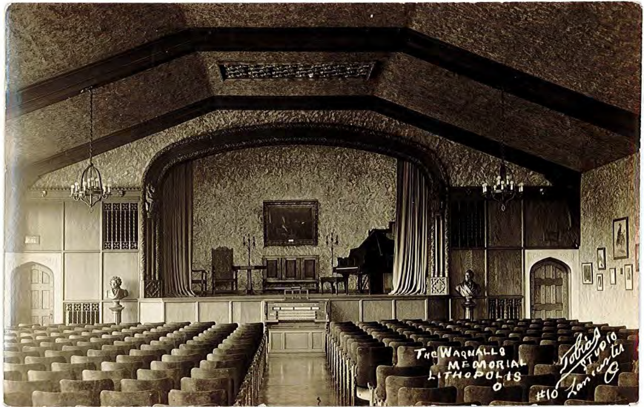
Figure 12: Interior of Auditorium in 1925 Memorial Building, pre-1960. Image courtesy of Wagnalls Memorial Foundation Archives.
