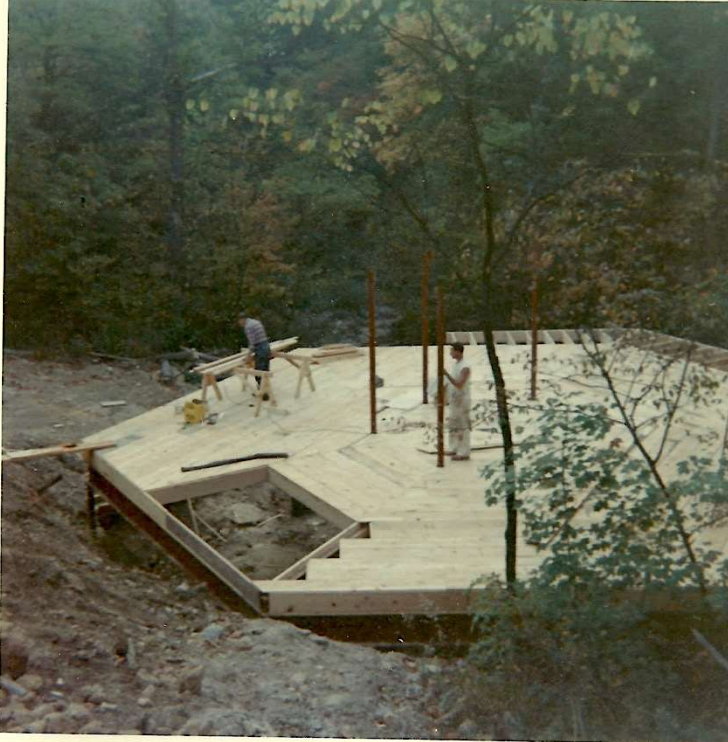
29 of 34: Construction of Dombar House and Studio: first floor. Circa 1967-68
