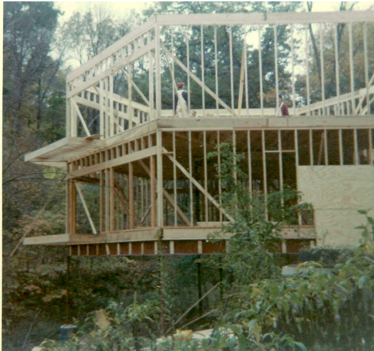
30 of 34: Construction of Dombar House and Studio: framing system. Circa 1967-68
