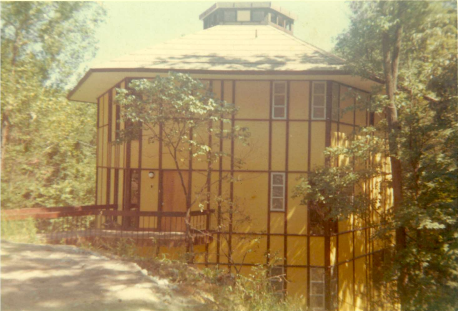
33 of 34: Construction of Dombar House and Studio: complete house from driveway. Circa 1968
