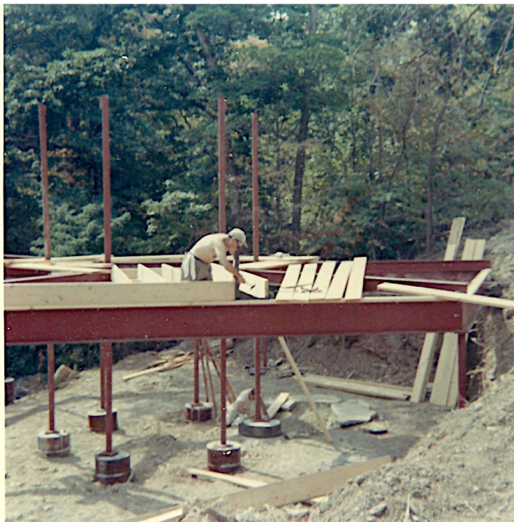
28 of 34: Construction of Dombar House and Studio: pier system. Circa 1967-68
