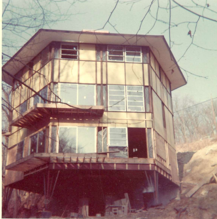
31 of 34: Construction of Dombar House and Studio: construction of balconies. Circa 1967-68
