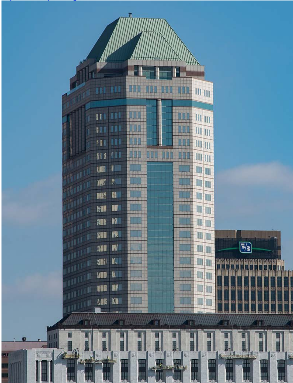
Figure 29. Vern Riffe State Office Building, 1988, 77 S. High Street. Source: https://en.wikipedia.org/wiki/Vern_Riffe_State_Office_Tower .
