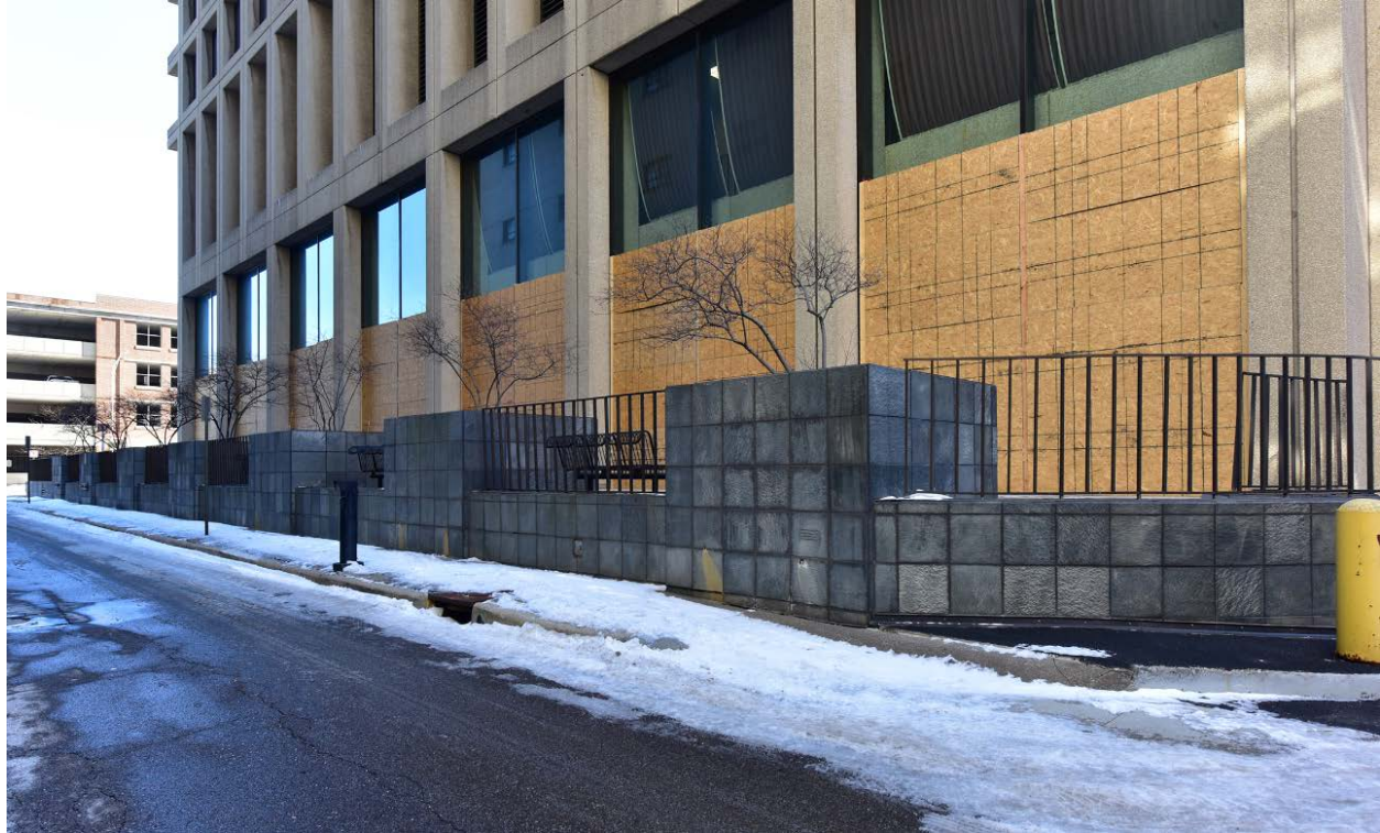
Figure 5. View looking southeast along the north side of the north plaza, showing quartzite veneer, planters, and railings. Source: Brad Finch, February 2021.
