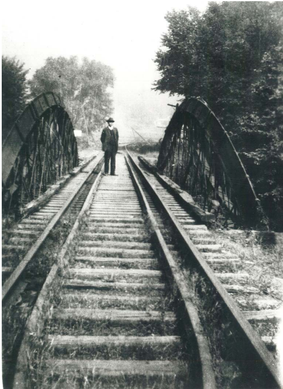
Figure 11: In 1859, Zenas King was still working for Moseley & Company in Cincinnati when this bridge was built over Storms Creek north of Ironton, in Lawrence County, Ohio, for the Iron Railroad, a line established to service charcoal iron furnaces. Ohio History Connection
