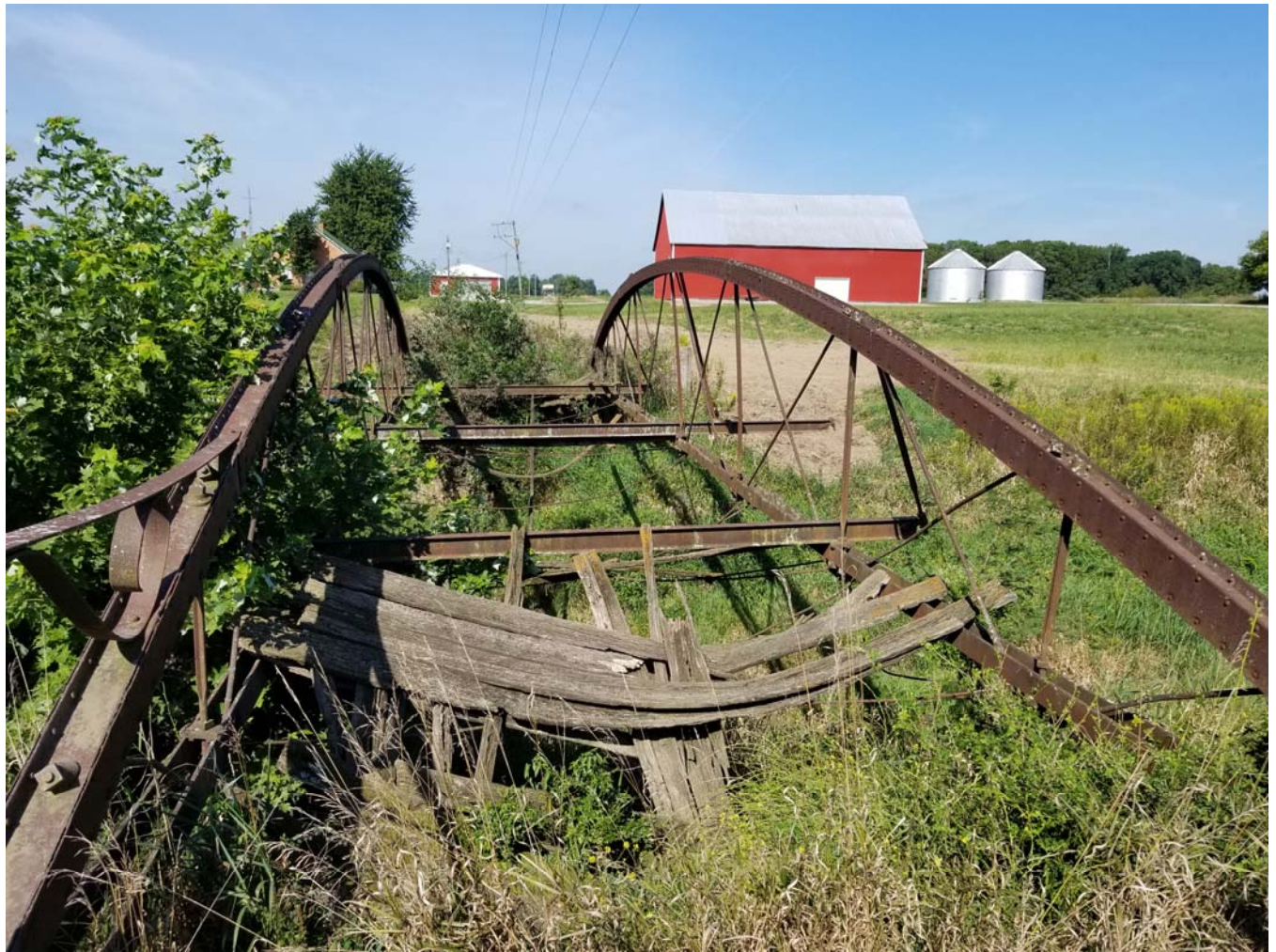
Figure 04: Overall condition, August 2020. Bach Steel Photo
