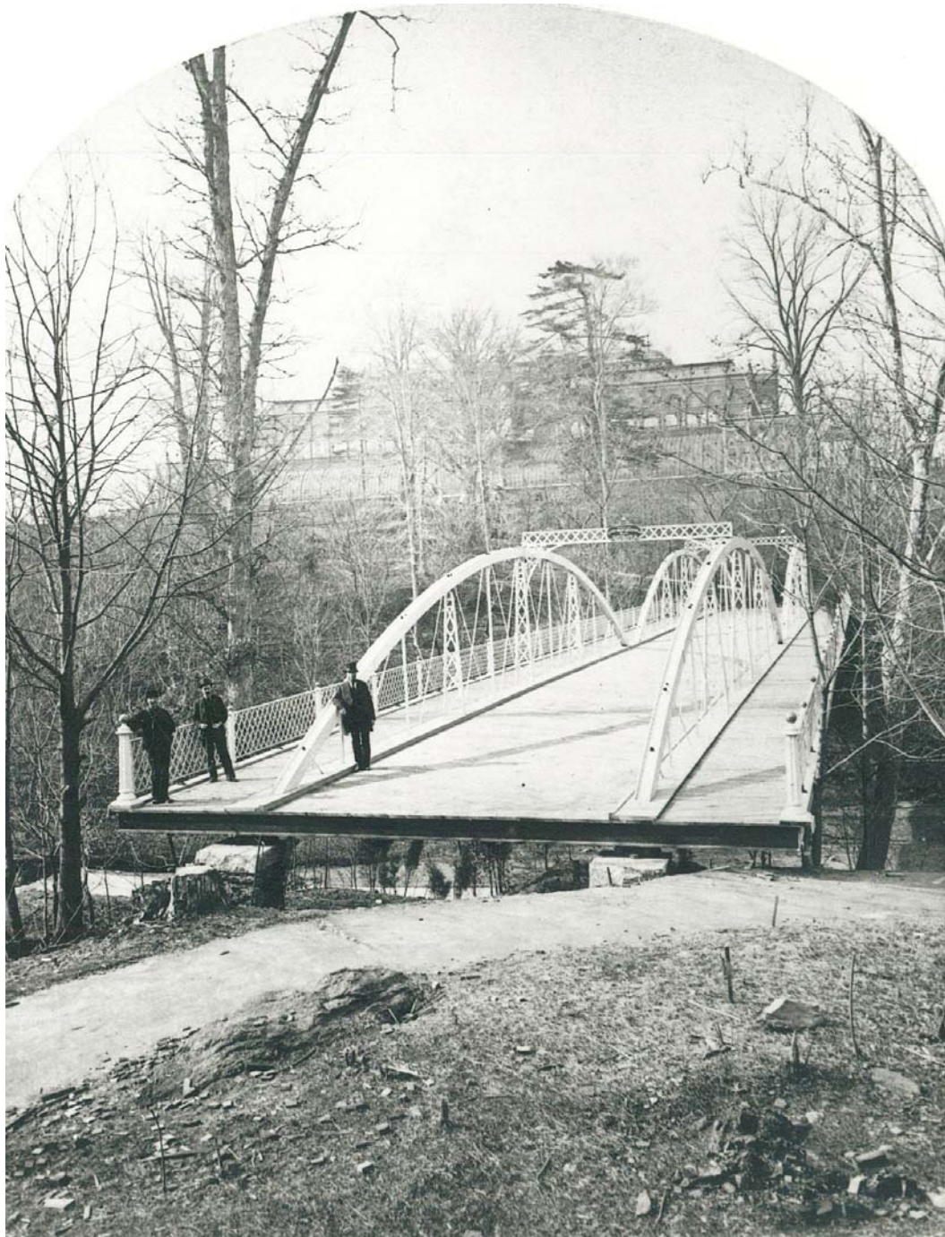
Figure 14: Evidence of the success of King's patent bowstrings was their choice for a prominent location in the Centennial International Exposition of 1876 in Philadelphia's Fairmount Park. Zenas King proudly stood at the end of the bridge upon its completion. Robert M. Vogel Collection
