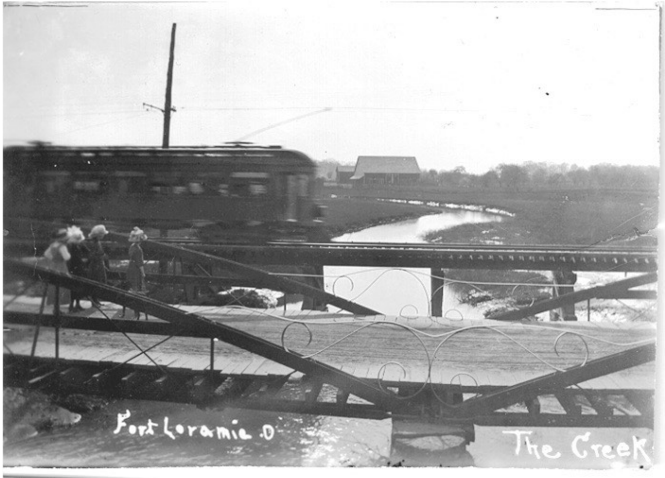
Figure 02: Historic view of bridge on original location, circa 1912. Ken Sowards Collection
