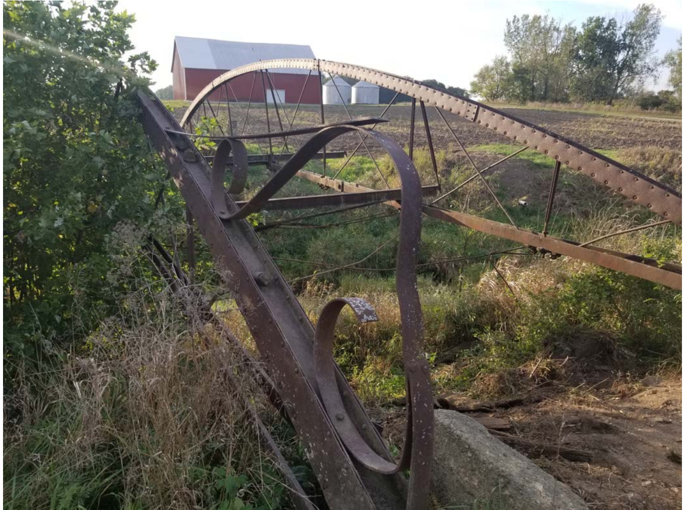
Figure 06: Condition of scrollwork approach, August 2020. Bach Steel Photo
