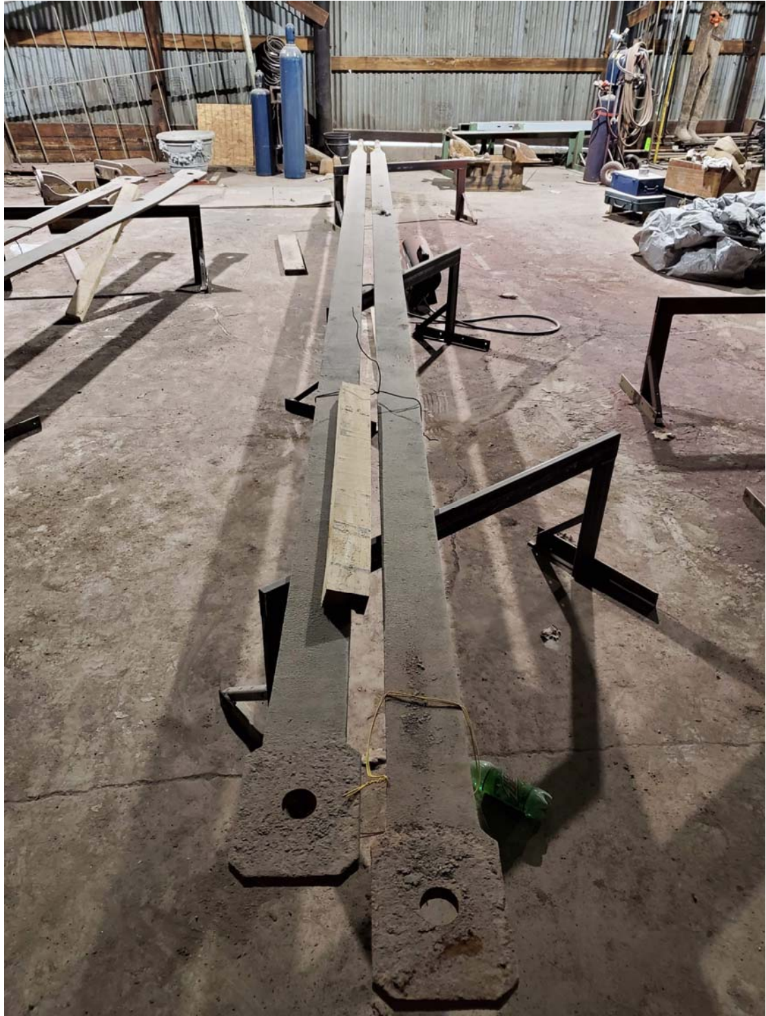
Figure 07: Pad welding repairs of eye bar “eyes.” Bach Steel Photo
