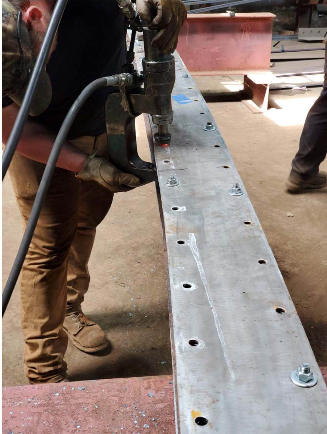
Figure 08: Riveting new side plate on tube. Bach Steel Photo
