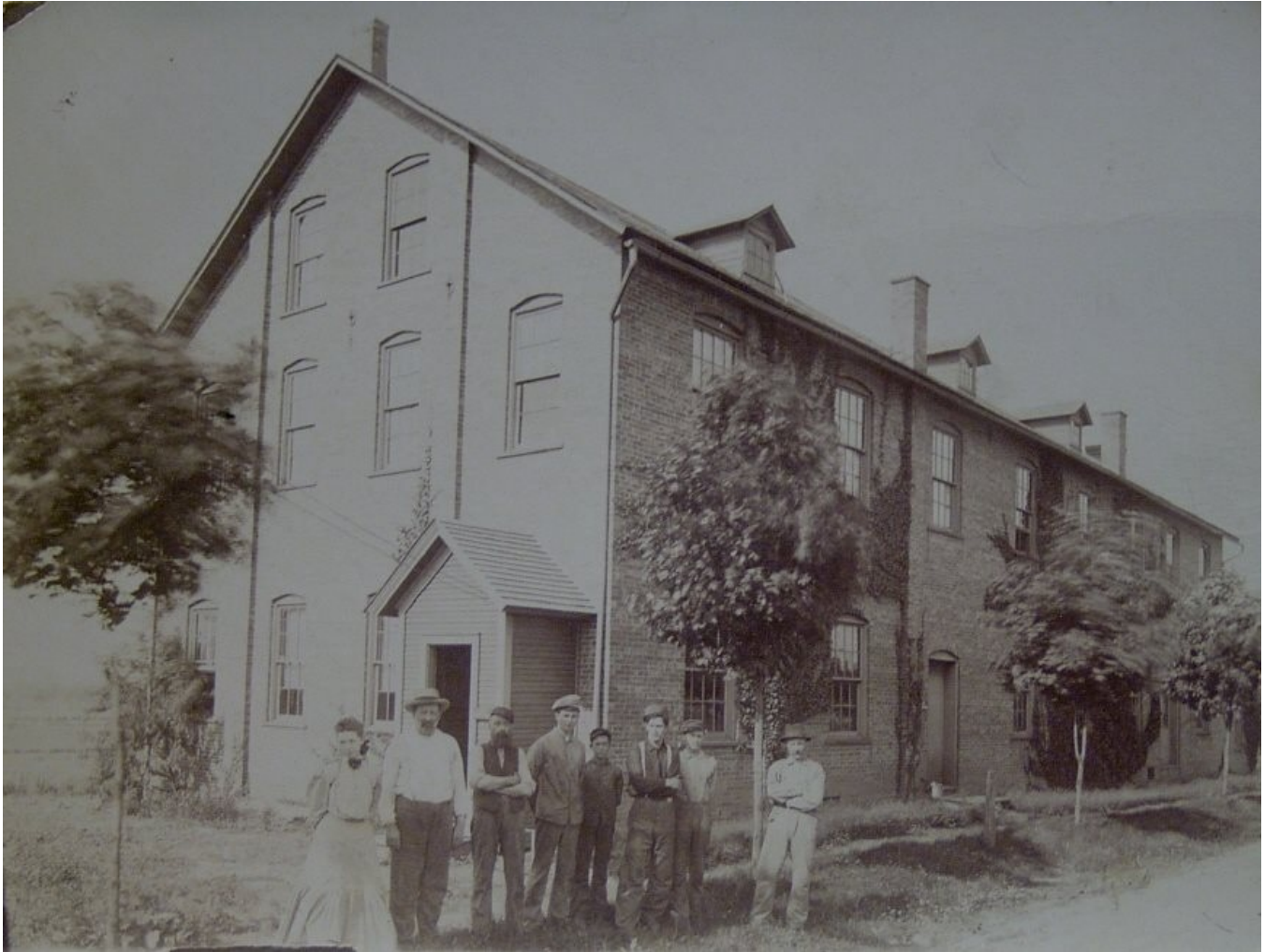
Figure 1: 1904 Schantz Organ Company factory building, undated (Abraham J. Schantz and employees). Courtesy of Schantz Organ company archive.
