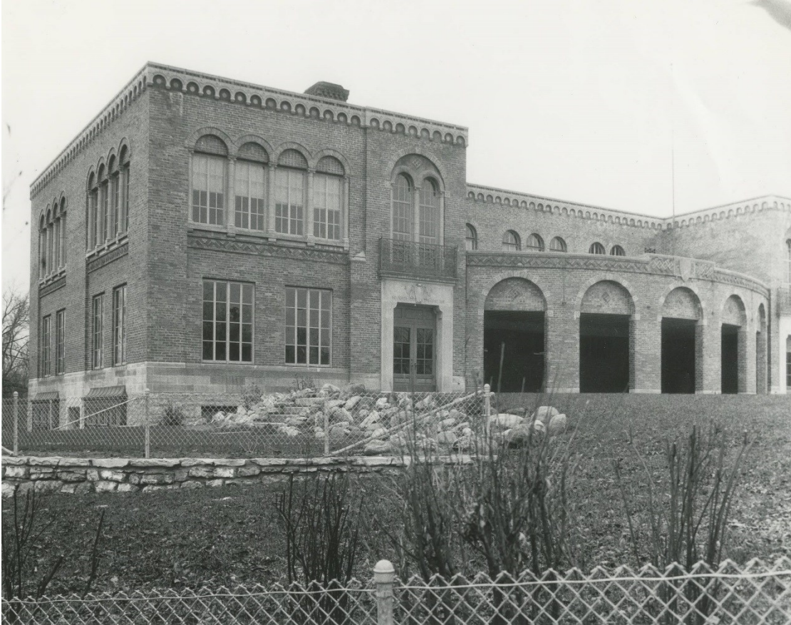
South and West Elevations 1928 Building Courtesy Columbus Metropolitan Library Historic Photograph Collection
