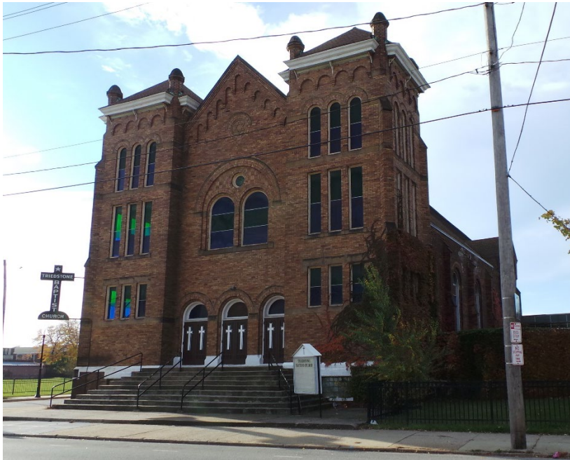
Figure 06. Temple designed by Albert Janowitz in 1905 for the Oheb Zedek congregation (now Triedstone Missionary Baptist Church) located at 3782 Community College Ave. (formerly E. 38 th street) Photo courtesy of Cleveland Restoration Society, 2022.
