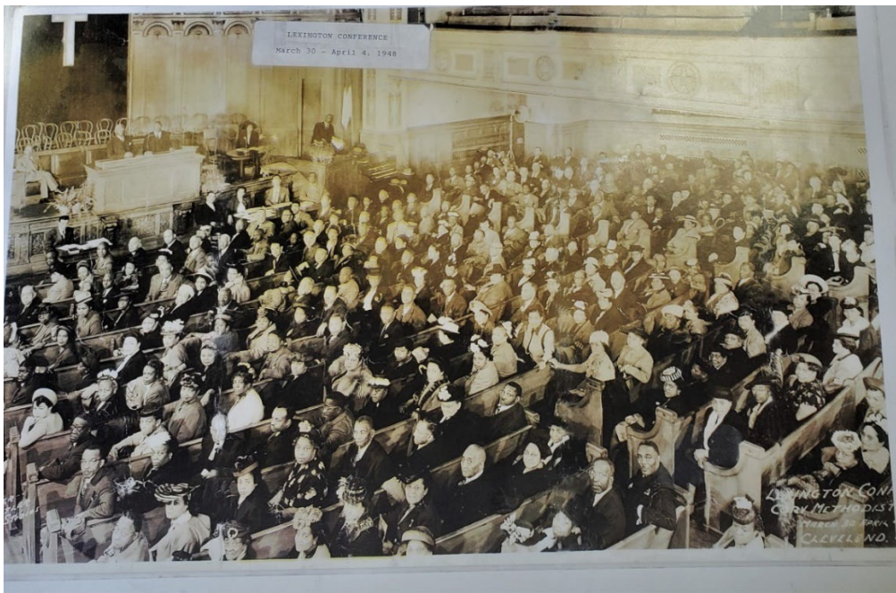
Figure 13. Lexington Conference, held inside the sanctuary at Cory United Methodist Church, 1948. Image courtesy of Cory United Methodist Church.
