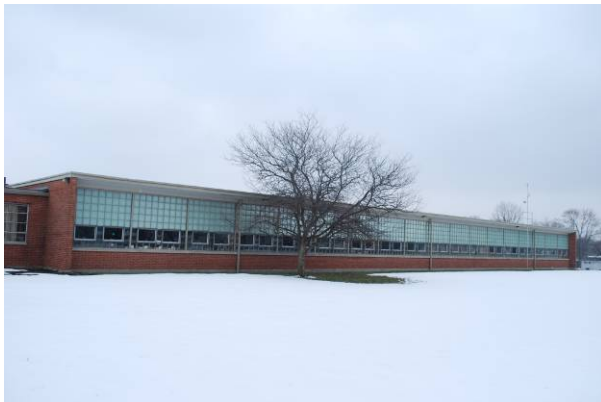
With wingwall Rolling Fields Intermediate School (1955) 2900 Acosta St., Kettering MOT-05490-06
