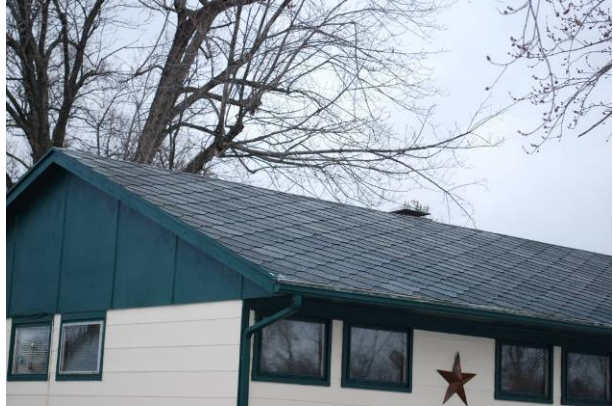
Patterned roof shingles
