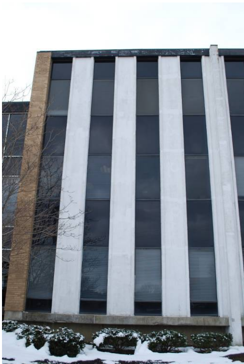
With vertical concrete panels Financial South Office Building (1968) 5335 Far Hills, Kettering MOT-05494-03
