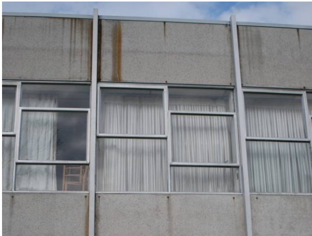
Extruded mullions Fairview Baptist Church (1965) 6401 N. Main St., Dayton MOT-05332-09
