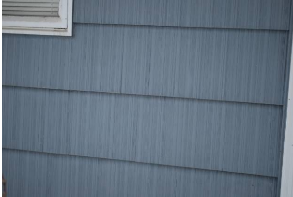
Wood grain siding
