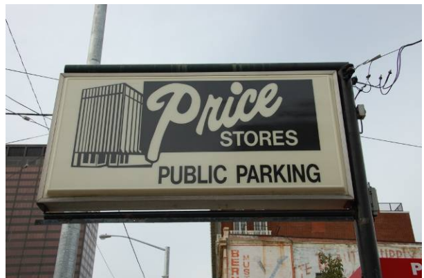
Plastic hollow core – pole mounted Price Stores (ca. 1950s) 50 S. Jefferson St., Dayton MOT-05298-15
