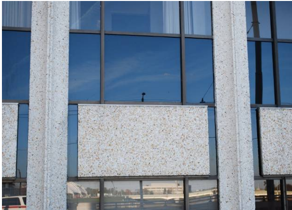
With exposed aggregate spandrel panels Beerman Building Annex (1967) 5 W. Monument Ave., Dayton MOT-05208-15
