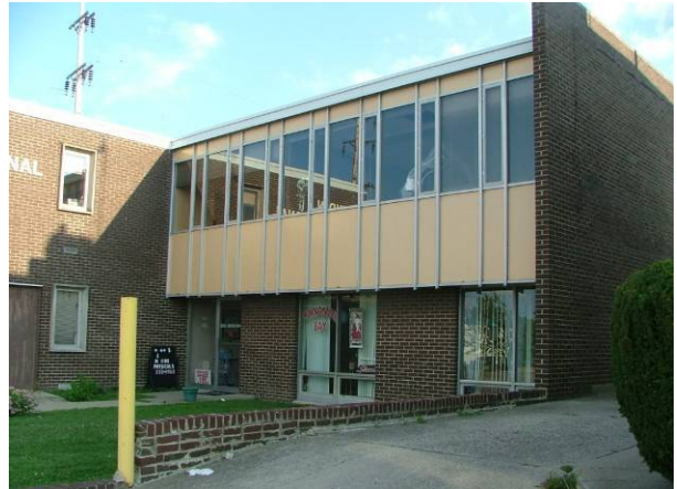
With porcelain enamel metal spandrel panels Linden Professional Building (1964) 2838 Linden Ave., Dayton MOT-05200-61
