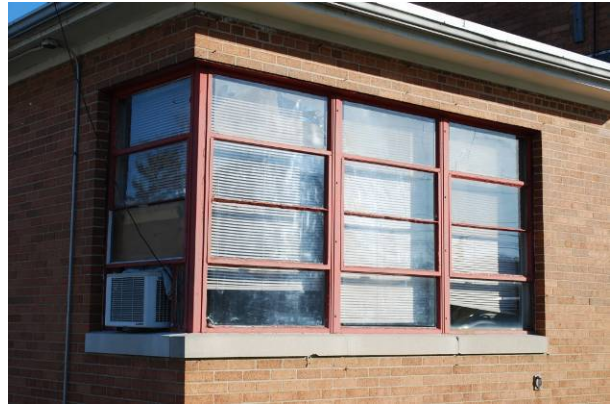
Turning corner Harrison Twp. Fire Station #94 (1958) 5190 Markey Rd., Dayton MOT-05337-09
