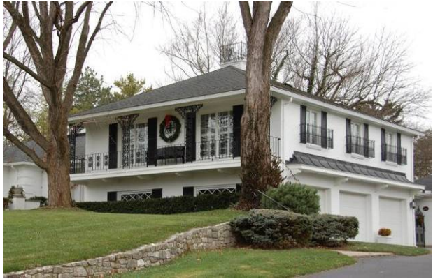
Balcony elements Richard Fisher House (1962) 5835 Kimway Dr., Dayton MOT-05564-03
