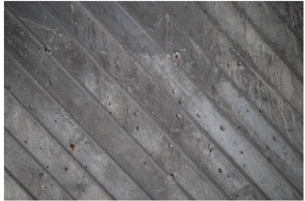
Decorative formed finish Kettering City Hall (1970) 3600 Shroyer Rd., Kettering MOT-05488-06
