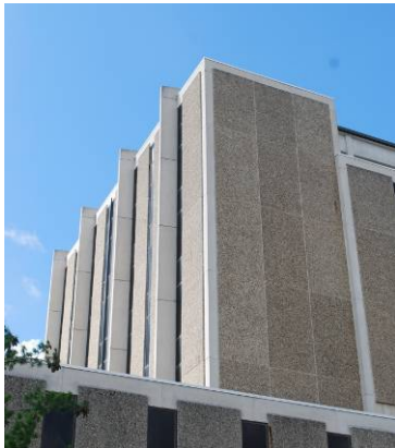
Curtain wall system Roesch Library, University of Dayton (1969) 300 College Park Ave., Dayton MOT-05158-60
