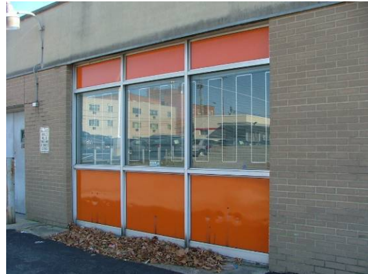
Spandrel panels Burroughs Corp. Business Machines (1964) 131 Salem Ave., Dayton MOT-05291-43
