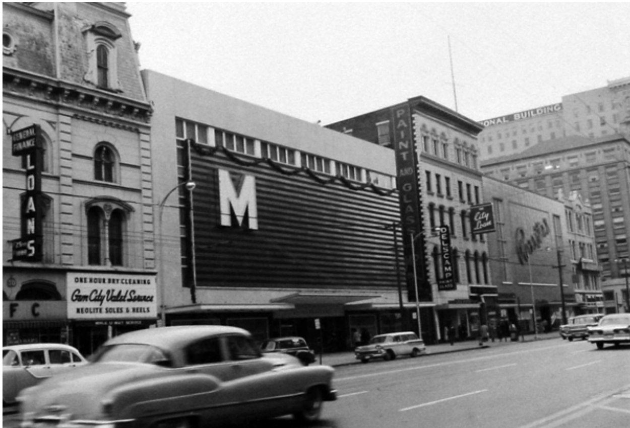
Metropolitan Building, 1959 (Historic Image 48)
