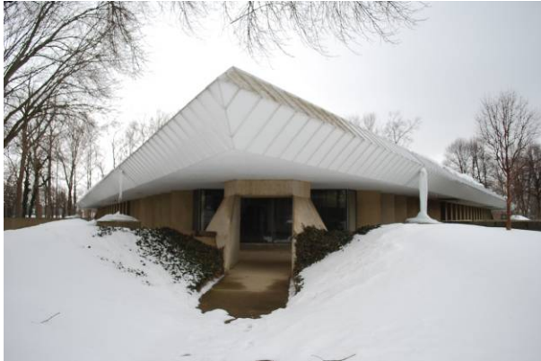
Continuous projecting - angled Kettering City Hall (1970) 3600 Shroyer Rd., Kettering MOT-05488-06
