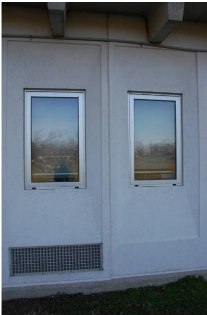
Formed concrete panels Wright Elementary School (1967-68) 480 W. Funderburg Rd., Fairborn GRE-01202-10
