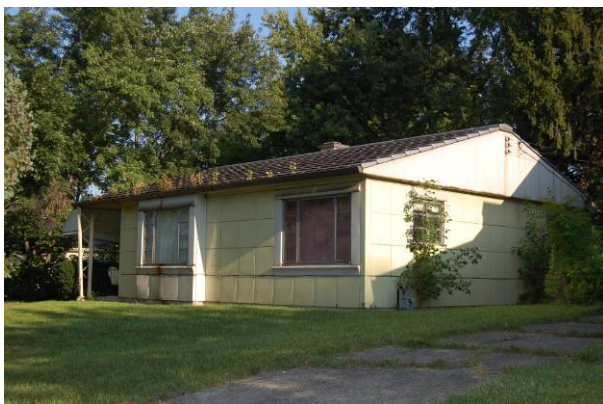
Panel cladding Chapman-Lustron House (1949) 3007 Cornell Dr., Dayton MOT-05162-38
