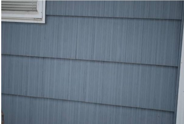
Wood grain siding
