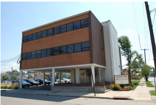
Pilotis with driveway
