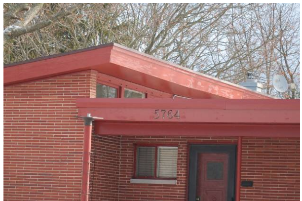
Above adjacent roofline 5764 Barbanna Ln., Trotwood (1955) MOT-05521-08
