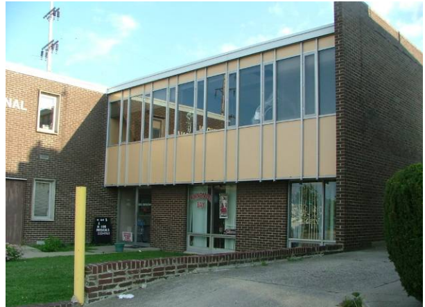
With porcelain enamel metal spandrel panels Linden Professional Building (1964) 2838 Linden Ave., Dayton MOT-05200-61
