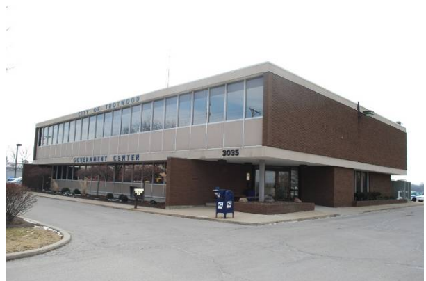
Spandrel of ribbon wall system Trotwood Government Center (1970) 3035 Olive Rd., Trotwood MOT-05469-08
