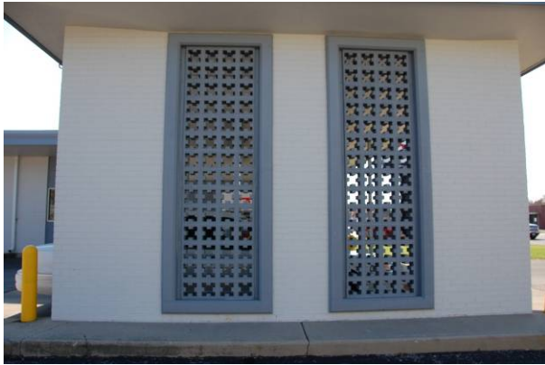
Screen integrated into façade Vandalia State Bank (1950) 4600 N. Dixie Dr., Dayton MOT-05407-09
