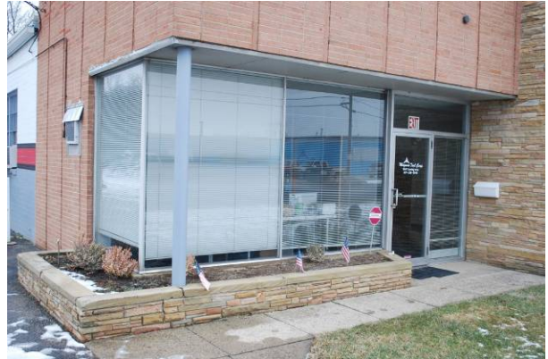
Corner recessed with storefront General Diaper Service (1955) 1407 Stanley Ave., Dayton MOT-05506-48
