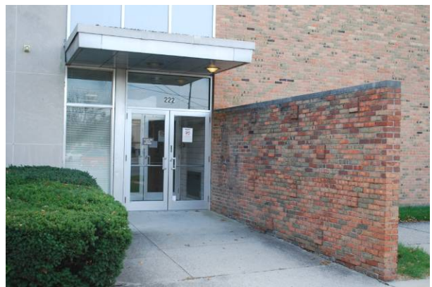
Wing wall at entrance State Employment Service (1959) 222 Salem Ave., Dayton MOT-05256-35
