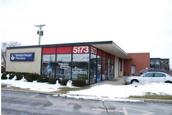
With porcelain enamel metal spandrel panels Brandt Medical Center (1963) 5173 Brandt Pike, Huber Heights MOT-05520-14
