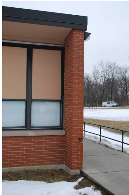
Brick stack bond Wayne High School (1959-75) 5400 Chambersburg Rd., Huber Heights MOT-05516-14
