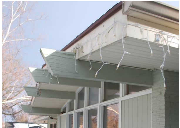
Exposed roof beams 396 Highland Terr., Kettering (1960) MOT-05545-06
