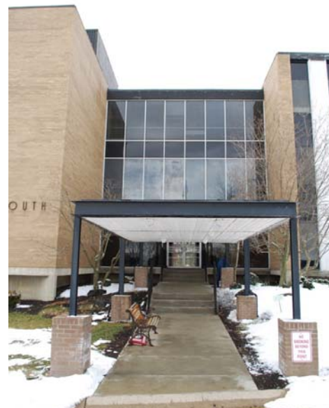
Recessed multi-story with canopy Financial South Office Building (1968) 5335 Far Hills, Kettering MOT-05494-03
