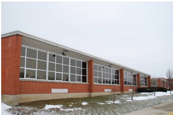
Multiple brick stacked bond Fairmont East High School (1962) 3000 Glengarry Dr., Kettering MOT-05491-06
