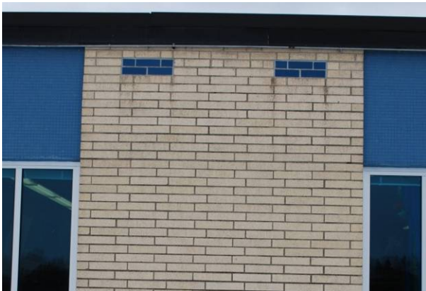
Elongated glazed brick with color accent John F. Kennedy Jr. High School (1967) 5030 Polen Dr., Kettering MOT-05496-06
