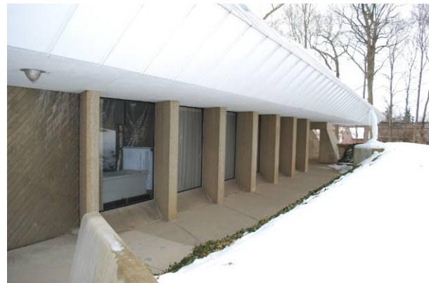
Angled concrete fins Kettering City Hall (1970) 3600 Shroyer Rd., Kettering MOT-05488-06
