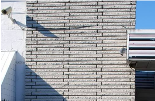
Elongated split face with offset bond Fox Cleaners & Laundromat (1947) 4333 N. Main St., Dayton MOT-05339-09
