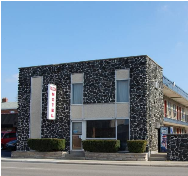
Lava rubble used as wall cladding Falcon Motel (1967) 36 N. Broad St., Fairborn GRE-01205-10
