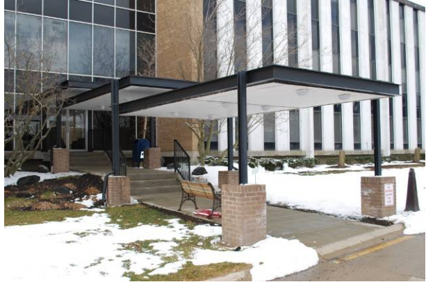
Stepped Financial South Office Building (1968) 5335 Far Hills, Kettering MOT-05494-03
