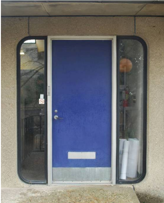
Eugene W. Betz, Architect office (1965) 2223 S. Dixie Hwy., Kettering MOT-05492-06
