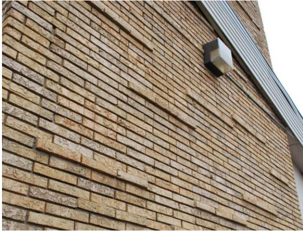
Elongated with offset bond and projecting pattern
