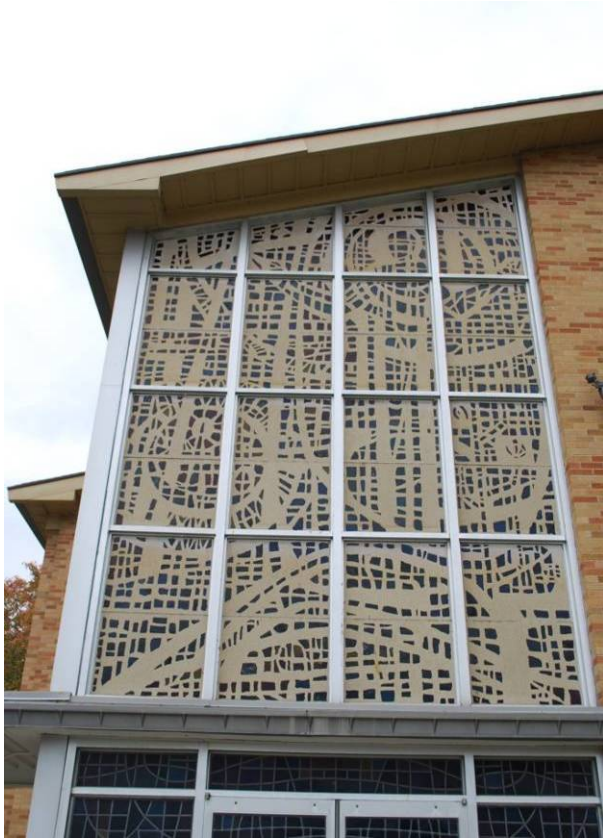
Dalle de Verre - curtain wall St. Rita's Catholic Church (1964) 5401 N. Main St., Dayton MOT-05335-09
