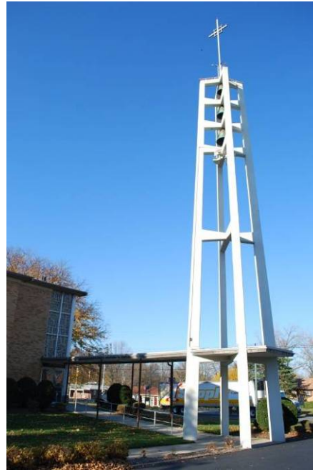
Bell tower with canopy
