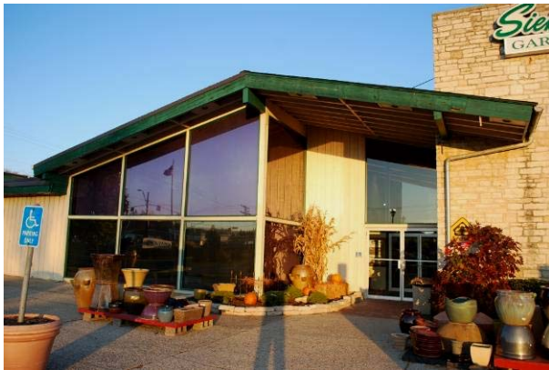
Low pitched gable with projecting eaves Siebenthaler Garden Center (1960) 6000 Far Hills Ave., Centerville MOT-05218-03
