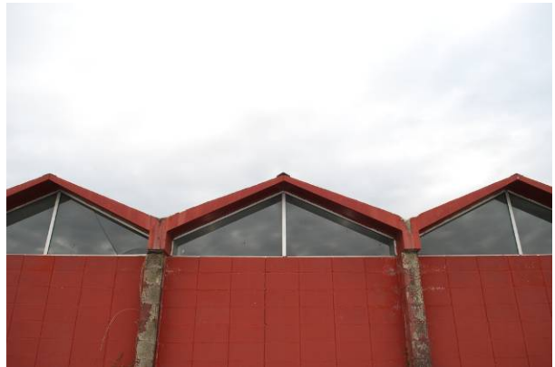
Angled Fill It Up Car Wash (1970) 5505 N. Main St., Dayton MOT-05334-09
