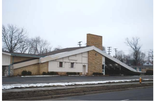
Low pitched gable with porte cochere Capri Motel & Coffee Shop (1956) 2700 S. Dixie Hwy., Kettering MOT-05498-06
