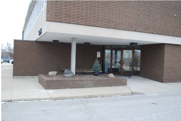
Corner recessed with planter and wing wall Trotwood Government Center (1970) 3035 Olive Rd., Trotwood MOT-05469-08
