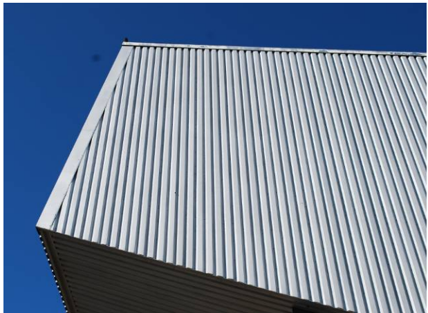
Vertical panel cladding University of Dayton Arena (1969) 1801 S. Edwin C. Moses Blvd., Dayton MOT-05157-64
