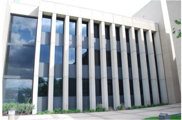
With piers Taylor Administration Center, Sinclair Community College (1967-72) 444 W. Third St., Dayton MOT-05202-15
