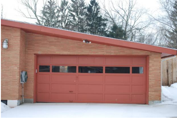
Residential garage door 220 Burgess Ave., Harrison Twp. (1960) MOT-05484-09
