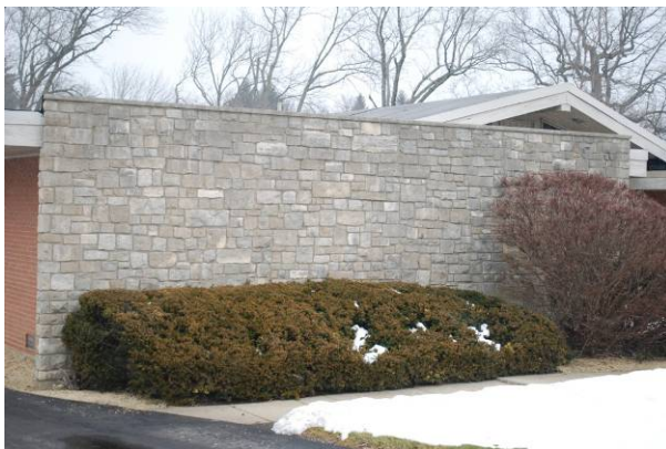
Side wall Greystone Medical (1965) 2033 E. Stroop Rd., Kettering MOT-05502-06
