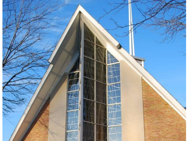
Prow - stepped Trinity Evangelical Lutheran Church (1963) 6540 N. Main St., Dayton MOT-05331-09
