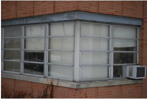
Continuous - turning corner General Diaper Service (1955) 1407 Stanley Ave., Dayton MOT-05506-48
