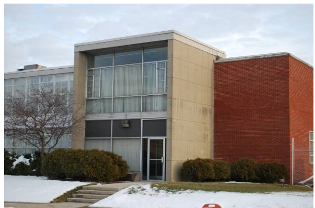
Vertical emphasis - projecting with concrete wing walls Globe Industries, Inc. (1954) 1784 Stanley Ave., Dayton MOT-05509-48
