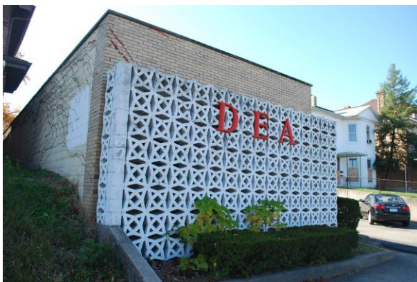
Standalone screen with signage First Finance (1964) 1013 N. Main, Dayton MOT-05344-44
