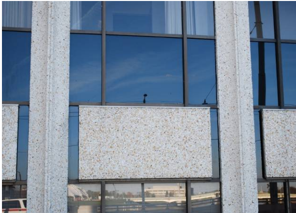
With exposed aggregate spandrel panels Beerman Building Annex (1967) 5 W. Monument Ave., Dayton MOT-05208-15
