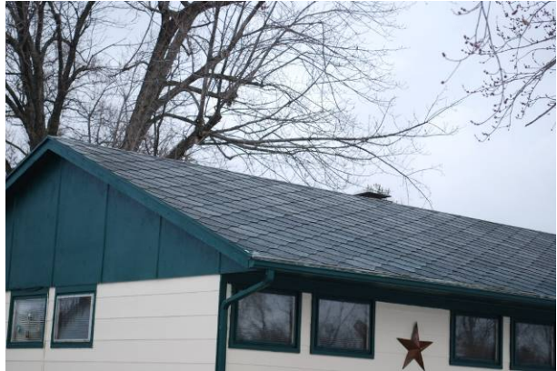
Patterned roof shingles
