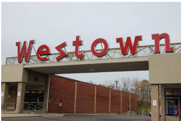
Plastic hollow core – individual letters Westtown Shopping Center (1957) 4227 W. Third St., Dayton MOT-05300-32
