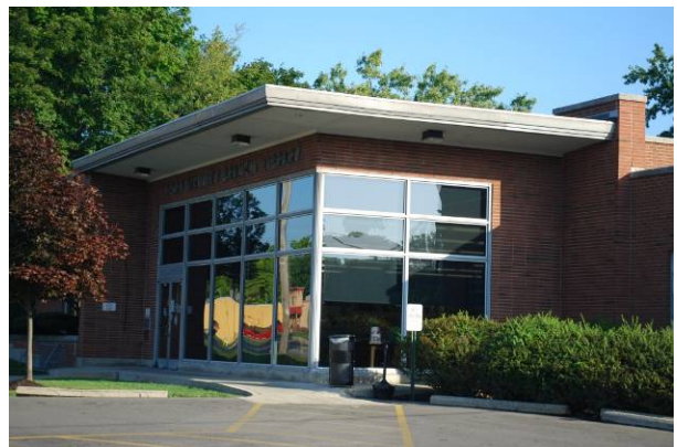
Corner projecting Ft. McKinley Library (1955) 3735 Salem Ave., Dayton MOT-05171-09
